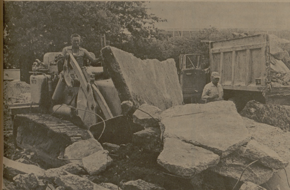
CRUNCH! A Caterpillar operator adds another slab of sidewalk to the scrap heap as workers continue preparations for building a lounge between dormitories 6 and 8 in the Duncan Area. Students gathered at hall windows and between the dormitories as the tractor methodically ripped up the concrete Tuesday. (Photo by Mike Wright)
