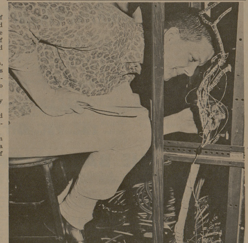
NEW ETV EQUIPMENT
