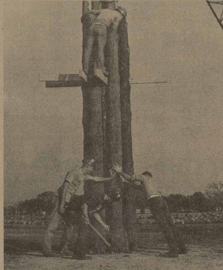
FIRST LOGS PLACED Juniors place the first series of logs around the center pole for the 1967 Bonfire. Behind them are some of the 1,100 logs that have been cut during the first half of the work period, which continues with cutting and stacking Sunday morning.
