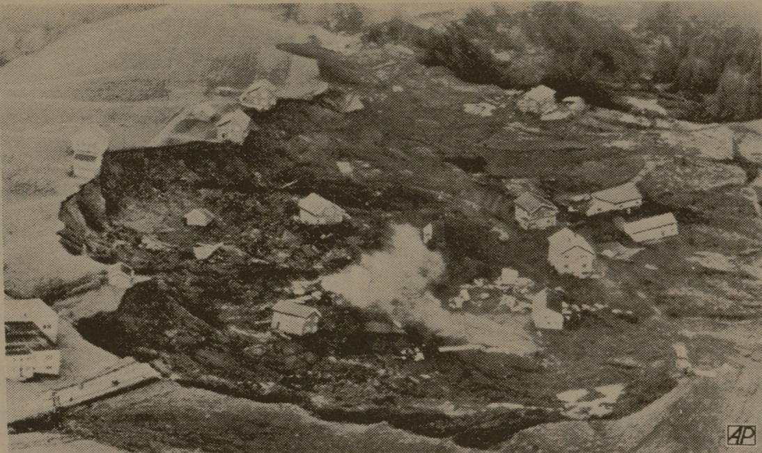
HOUSES TUMBLING BY NORWEGIAN LANDSLIDE Aerial view shows damage caused by a landslide at Troegstad in eastern Norway. Four persons were reported missing and 10 houses damaged or destroyed in the slide following torrential rains in the region. (AP Wire- photo by cable from Oslo)
