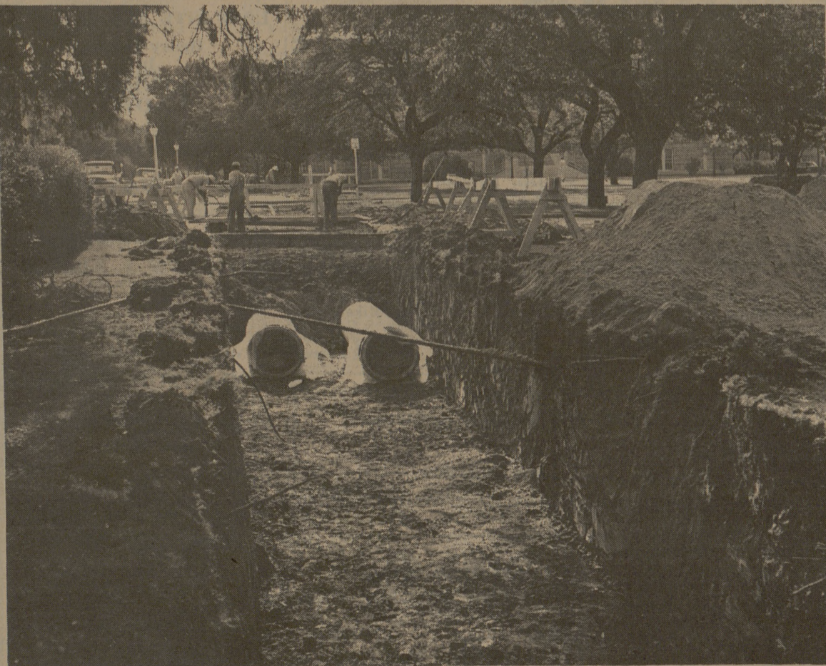
EXCAVATIONS FOR PIPELINE REACH SBISA
