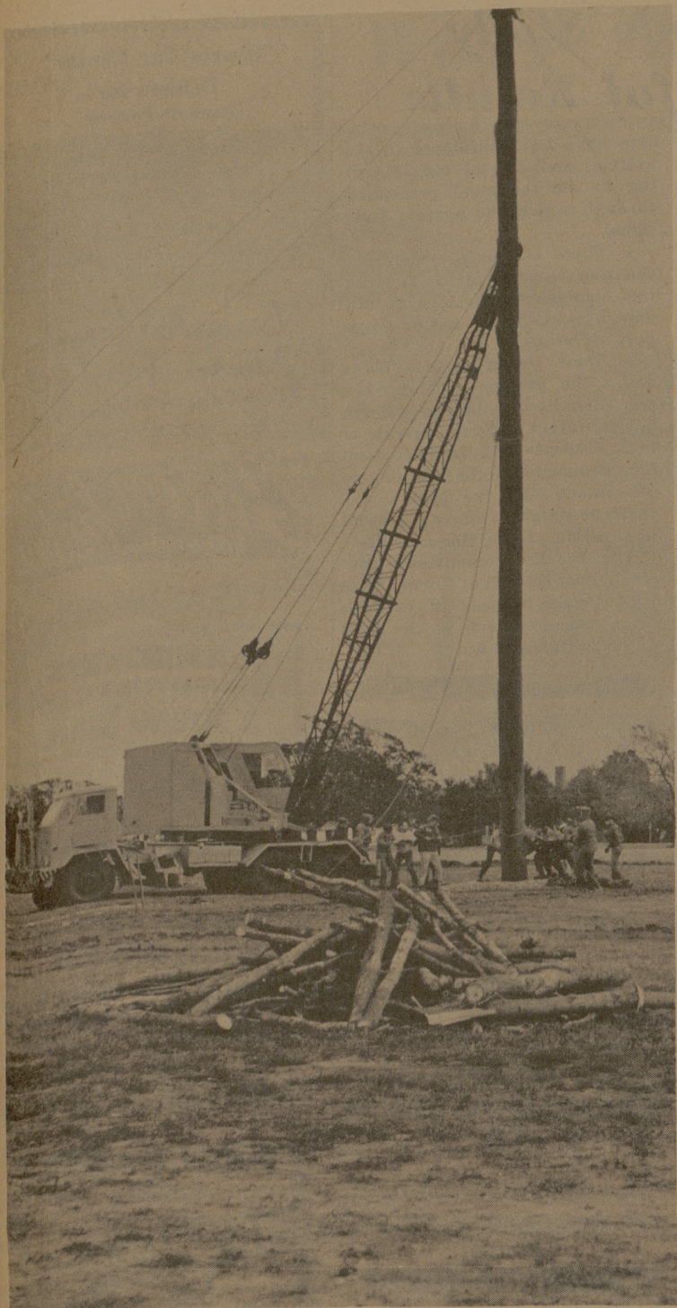
FOUNDATION COMPLETED ... for world's largest blaze.
