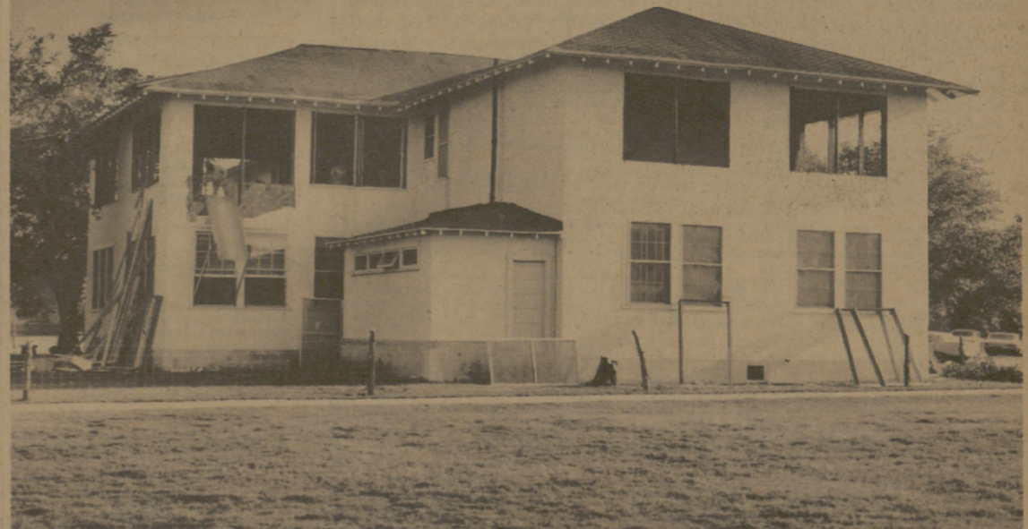
ON ITS WAY DOWN ... Music Hall now houses demolition team.
