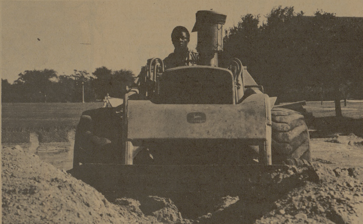
Parking Lot Renovation Begins
