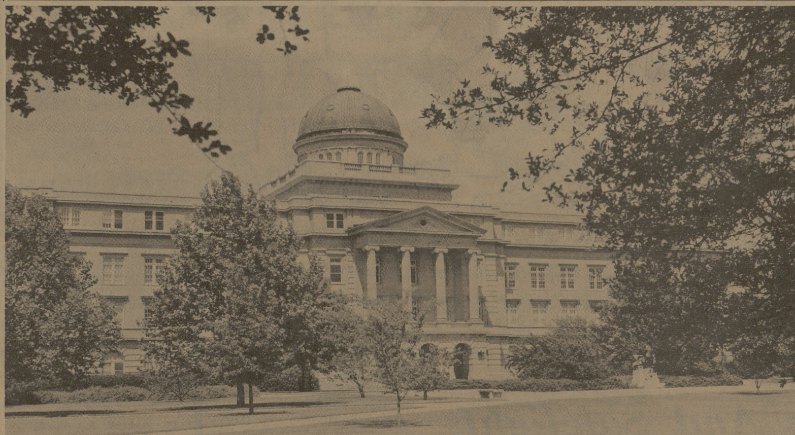
VIEW OF THE ACADEMIC BUILDING ... probably students have attended more classes in this famous Aggieland landmark than in any other building on campus.
