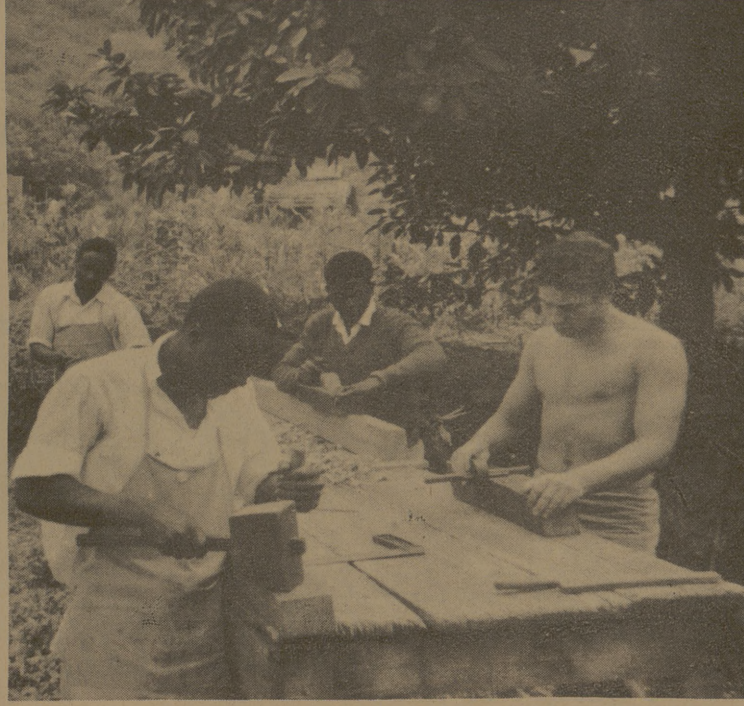
UGANDA WORKERS CONSTRUCT HOSPITAL American students helped build African project.
