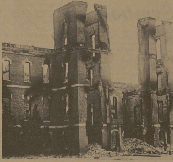
ONLY THE WALLS REMAINED Fire destroyed the building in 1912.
