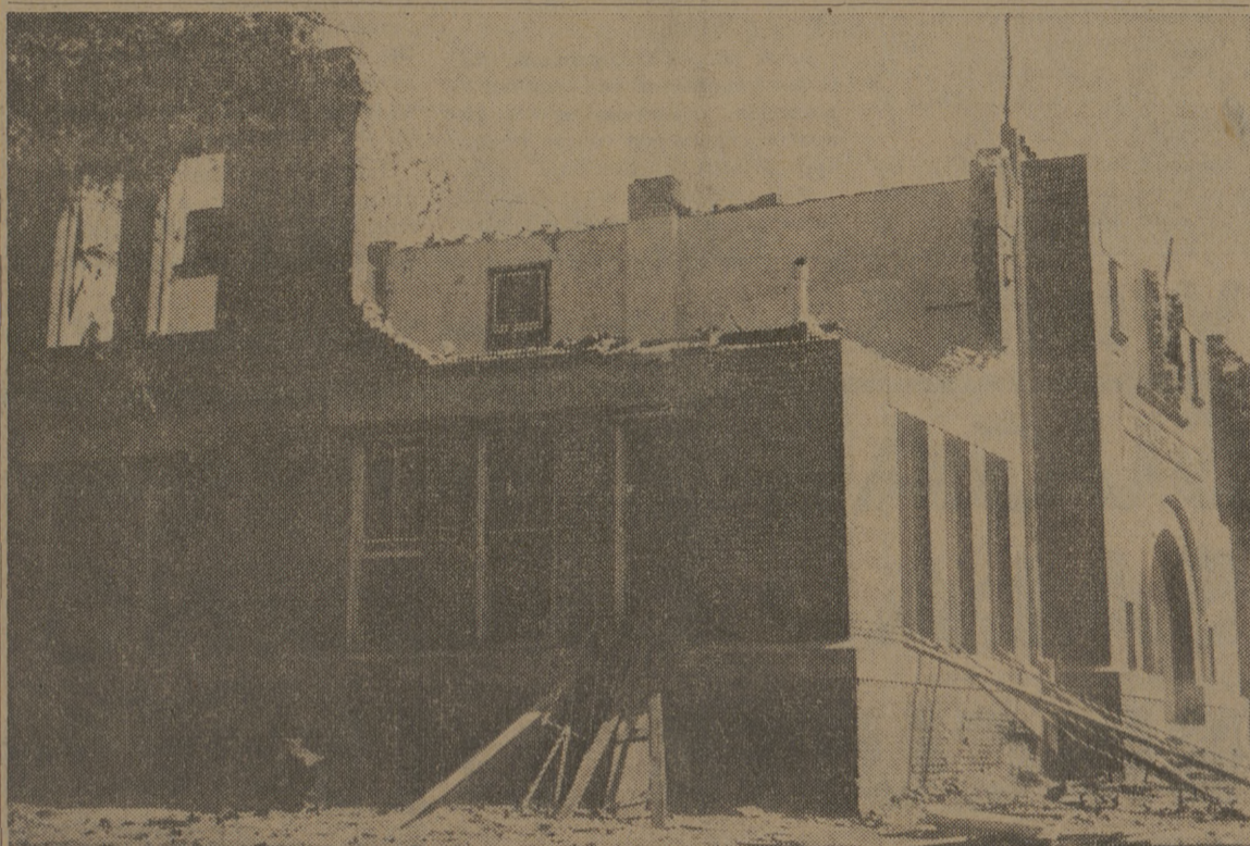
Landmark Being Demolished
