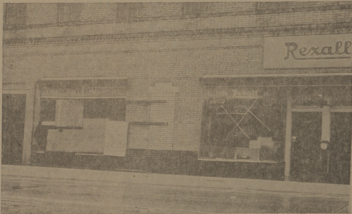
"Boards Replacing Glass"
