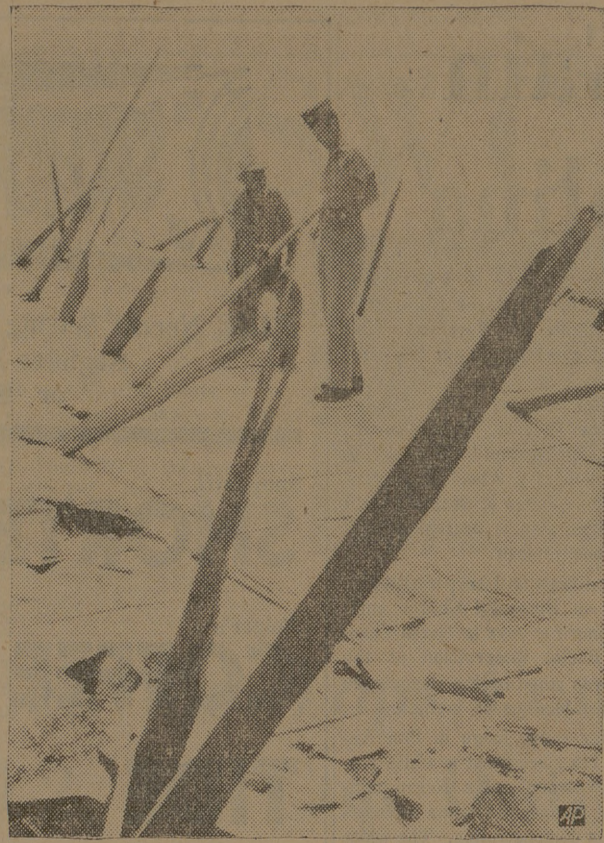
Debris Punctures Roof
