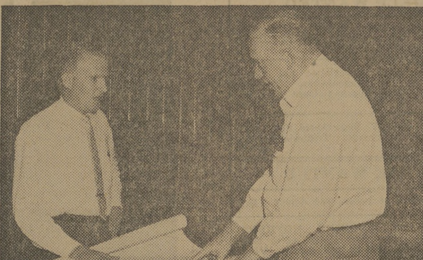
"8:30 a.m. I meet with one of our Foremen at the plant garage to discuss a cable-pressurizing job. We're putting all aerial cable in Hutchinson under air pressure to keep out moisture which causes cable failure and costly service interruptions."
