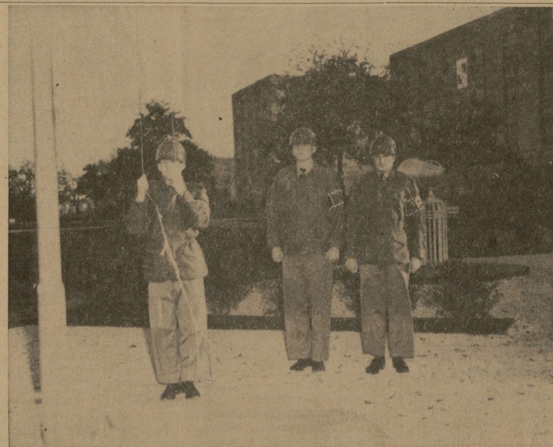
Area Around Flagpole Renovated
