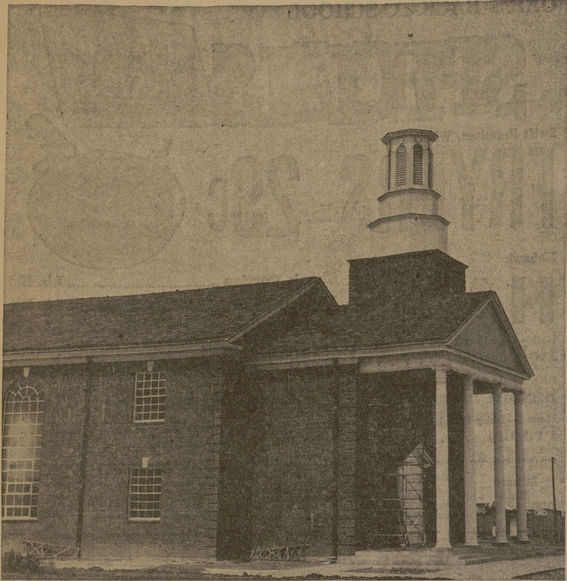
Chapel Nearing Completion
