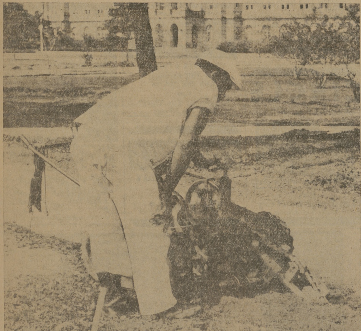
Workmen Install Lawn Sprinklers
