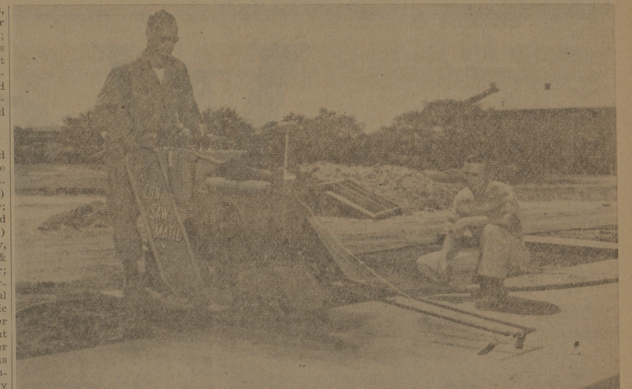
SAWING CONCRETE IS NO TROUBLE for this machine operated by John Tipton, whose company makes the cutter. The tool is being used for student observation and research information by the Civil Engineering Department. Watching the machine at work on the right is Bob M. Gallaway of that department.
