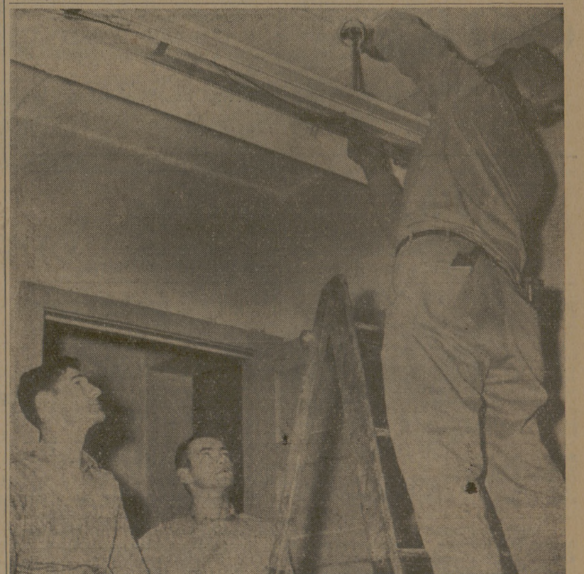
PUTTING THE FINISHING touches on the Journalism Department soon to be located on the ground floor of Nagle Hall is Tom Shaumfield, shown installing a fluorescent light. Watching with interest are (left to right) Warren R. Simmons and John Jefferson.
