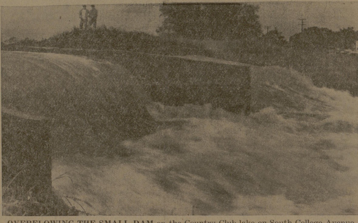
OVERFLOWING THE SMALL DAM on the Country Club lake on South College Avenue, water gushes out into the street to cut down traffic as shown in the pictures on each side. At 1:30 p.m. the lake level was about two feet below the top of the dam but by 2:30, it was well on its way out of the lake. Even then the spillway did not provide a big enough outlet as the water also overflowed the north end of the lake and spilled out on the highway.
