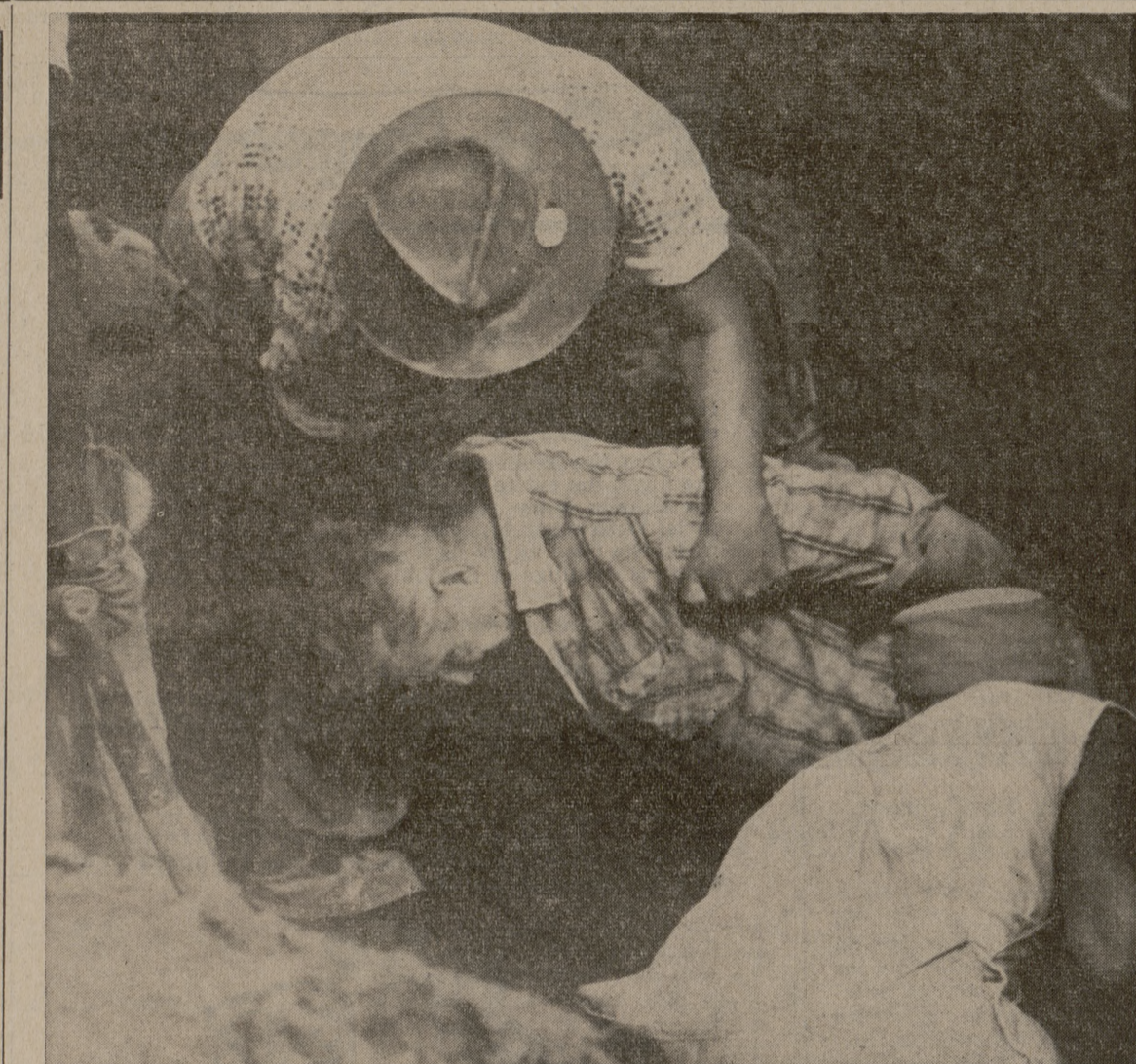
STILL TRAPPED by the sticky mud around his legs is Al Hambrick, labor foreman of the Lufkin Construction Company. Workmen are shown trying to pull him free from the wet dirt which crashed from the sides of the storm sewer ditch under construction near the Power Plant.
