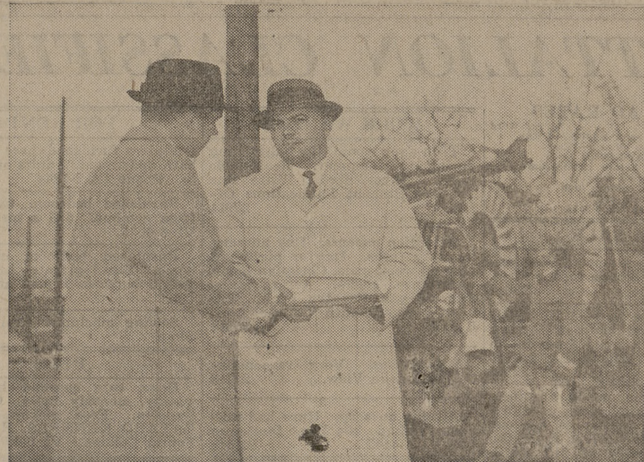
Ken Boekeloo (center foreground) at the scene of a cable installation project in Detroit.
