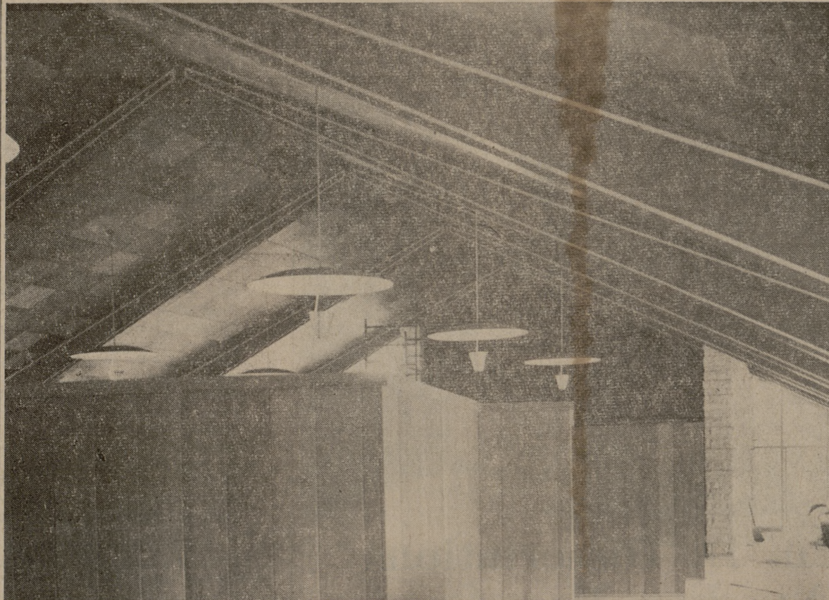
A BEAUTIFUL INTERMINGLING of spirituality and modern architecture is taking its final form in the $250,000 Inter-faith Chapel. The modern touch is evident all of the way from the floor to the inlaid ceiling and simplicity is heightened by the strength of the steel supporting beams.
