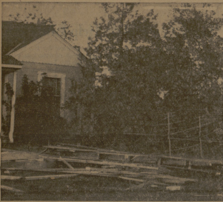
NO TELEVISION TONIGHT —One of the most often hit "victims" of the tornado were television antennas. Very few antennas in the path of the funnel survived being either torn off or bent over. The above antenna came down with part of the roof.
