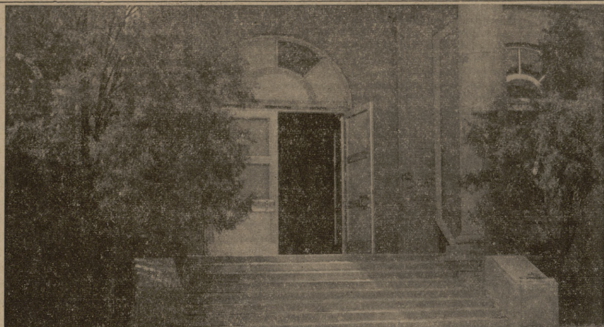
TO HOLD AGGIES IN —Aluminum doors are just a part of the face-lifting that Sbisa Hall is now undergoing. In addition the building is getting a new, low ceiling, a new ventilation system, and a multiple speaker public address system. Work will be completed by the beginning of the fall term.
