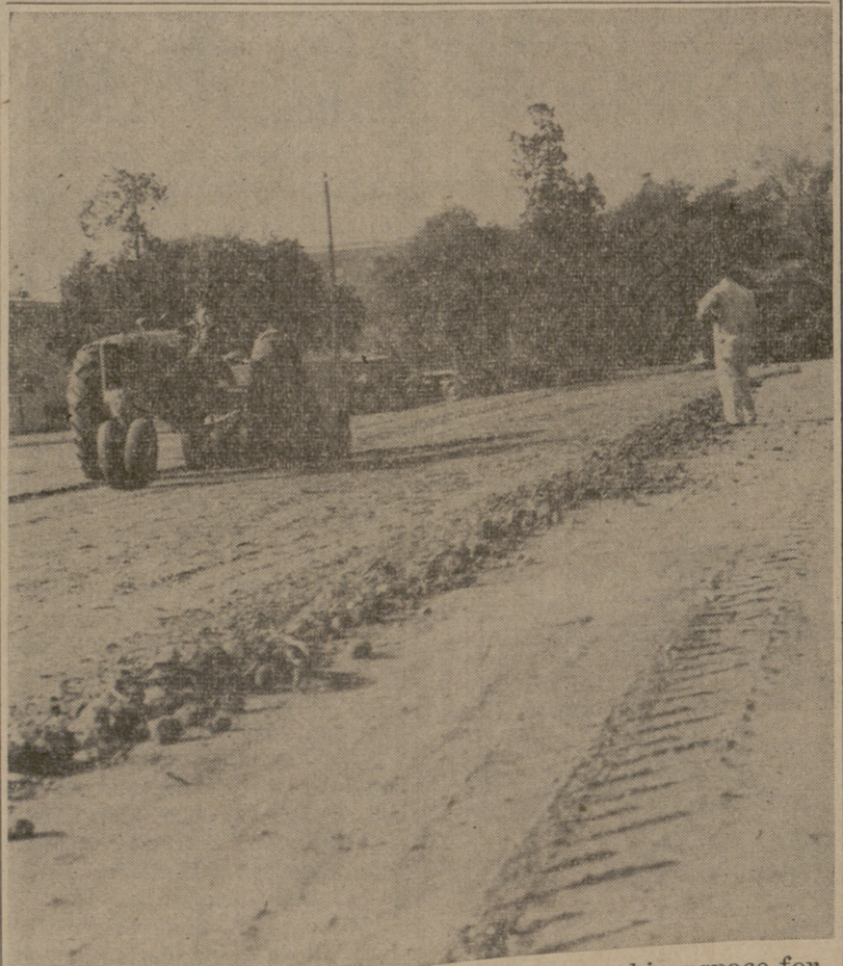
MORE SPACE —Workmen prepare more parking space for A&M students. This lot will be an extension of the Law-Puryear parking lot.
