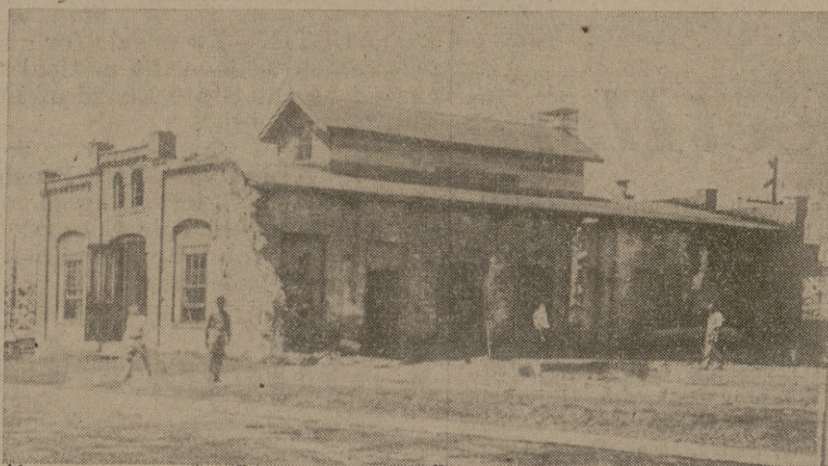
WHAT'S LEFT —The blacksmith shop, which was on the east side of the Mechanical Engineering building, was saved and used as a temporary shop. The shop was set up by R. W. Downard, assistant professor of mechanical engineering.
