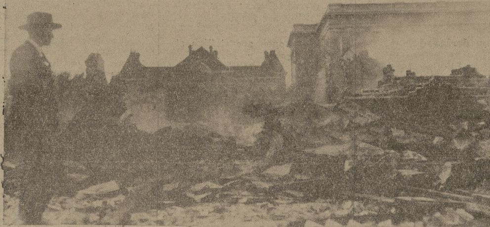
REMAINS —This is the remains of the old Mechanical Engineering building which burned on Dec. 6, 1921. The building and most of the equipment and other materials were destroyed. The Electrical Engineering building and Ross hall are shown in the background. The blurred area in the photo is smoke.
