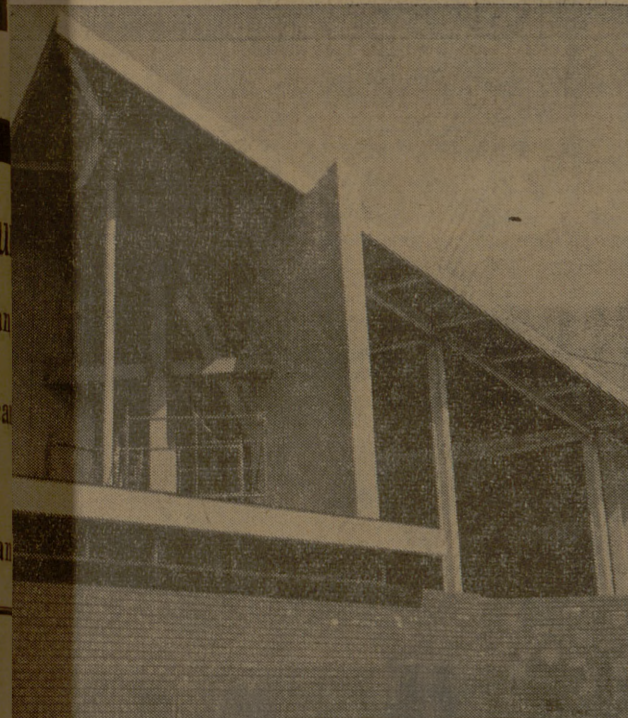
The new contemporary design Lutheran church in the corner of Cross and Tauber streets at North College Station, which was begun in January, will be the first of September, according to the Rev. Ernest Gert, pastor. The church, designed by Ernest Frank Lawyer, will seat 255 persons.
