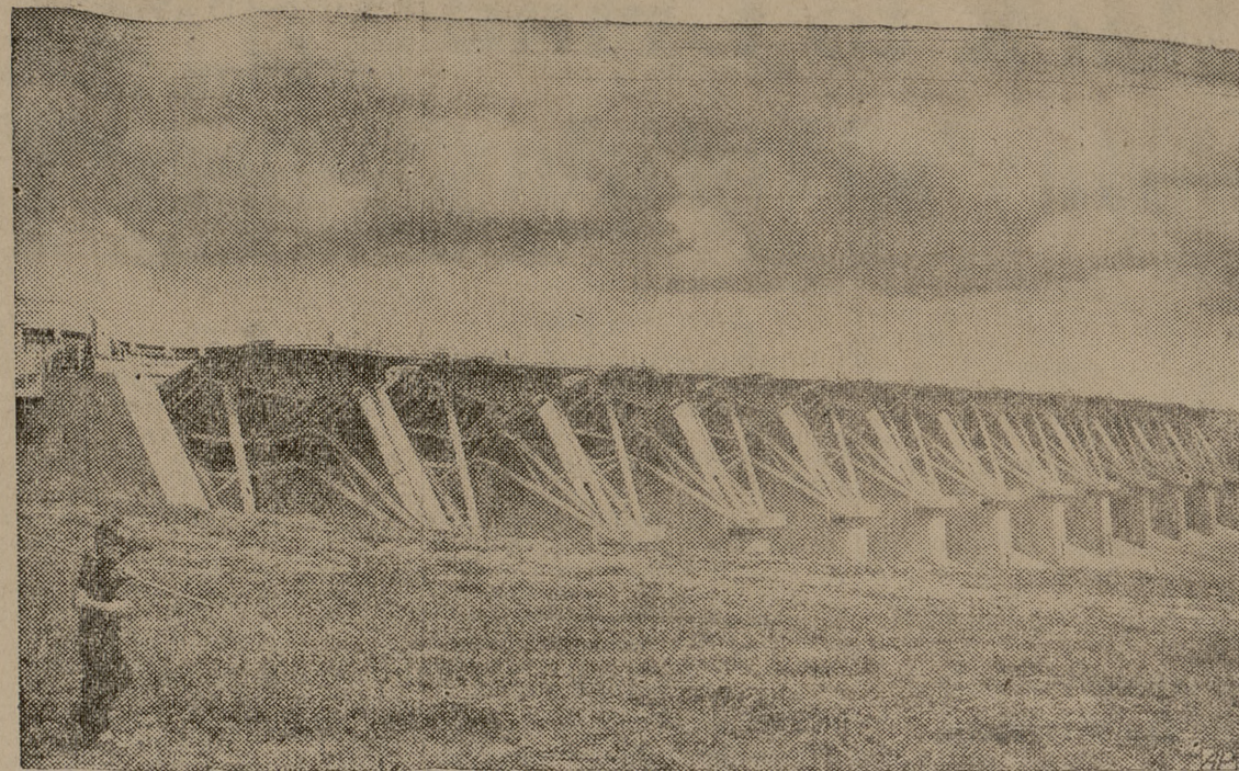
NEW DAM PROJECT —These 12 steel gates will soon be used to hold water at the New Lavon dam, located on the east fork of the Trinity river, near Wylie. The dam is a project of the Fort Worth district, Corps of Engineers. At left is Clinton Rabb, 5, of Wylie, waiting with his fishing tackle.
