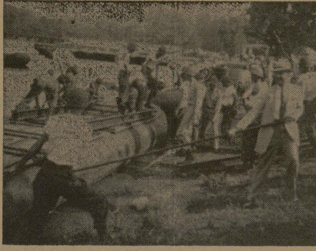
President M. T. Harrington gives a hand to this project at Ft. Belvoir, Va. as he takes part in an inspection tour of troops at the camp who are currently undergoing Summer training there in the Engineer ROTC. Men working on the pontoon bridge are from A&M and Penn State.
