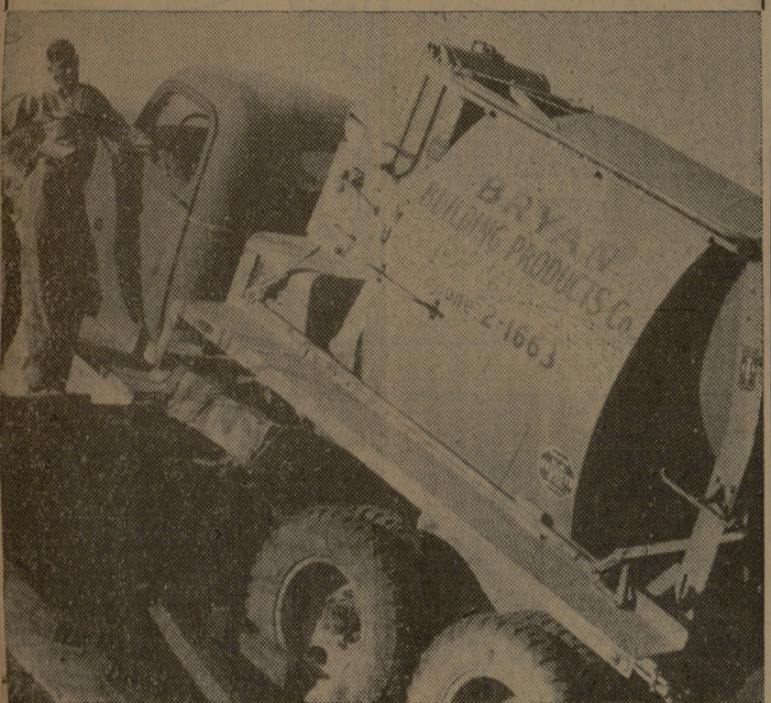
"It just kinda slid back . . . seemed like it would never get to the bottom." That was the only comment of Marvin Brinkley, Bryan truck driver whose 45,000 lb. cement truck fell through a wooden bridge just off the Airport Road late yesterday afternoon. Total damage: one bent drive shaft, a "shoved-up" gas tank and the cost of a drag-line to remove the truck. Brinkley, incidentally, was hauling cement for a bridge being built on the Butler property west of the campus.
