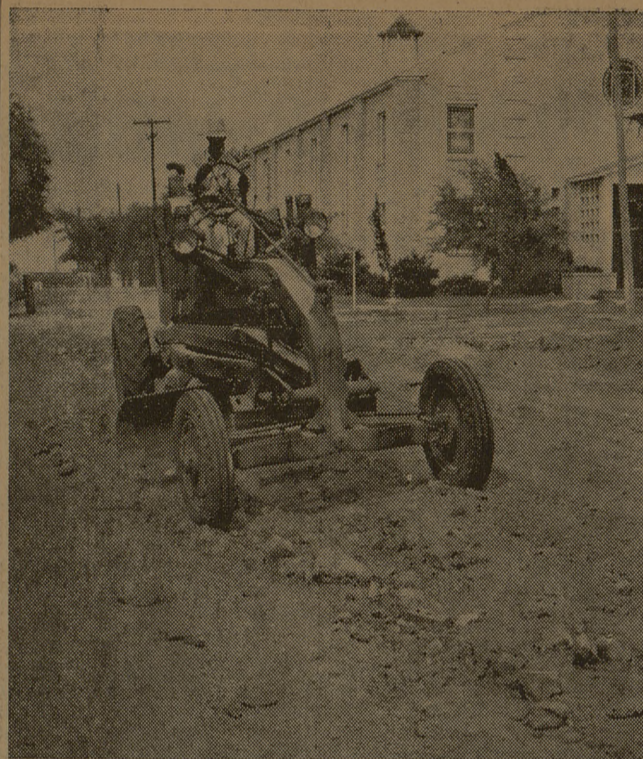
With hopes that no more drainage problems will cause people at the Church Street - Main Street intersection any more trouble, the city is currently grading and cutting down the level of the street and ditches so near flood conditions will not exist at this spot everytime a large rain falls.
