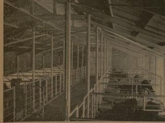
Part of the newly constructed \$100,000 Beef Cattle Center is the feeding shed with 31 dirt-floored stalls. Each stall contains an individual metal feeding box. A concrete water trough is con-structed under every other dividing fence between the stalls, half of the trough extending into each adjoining stall.
