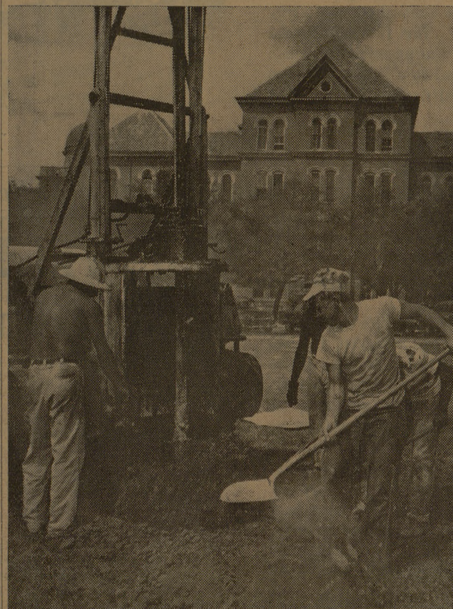
In the first step toward construction of the new college administration building, test holes have been drilled on the building site to determine depth of footings for the building. The new administration building will be located on the area just north of Goodwin Hall, across the street from the south side of the YMCA.
