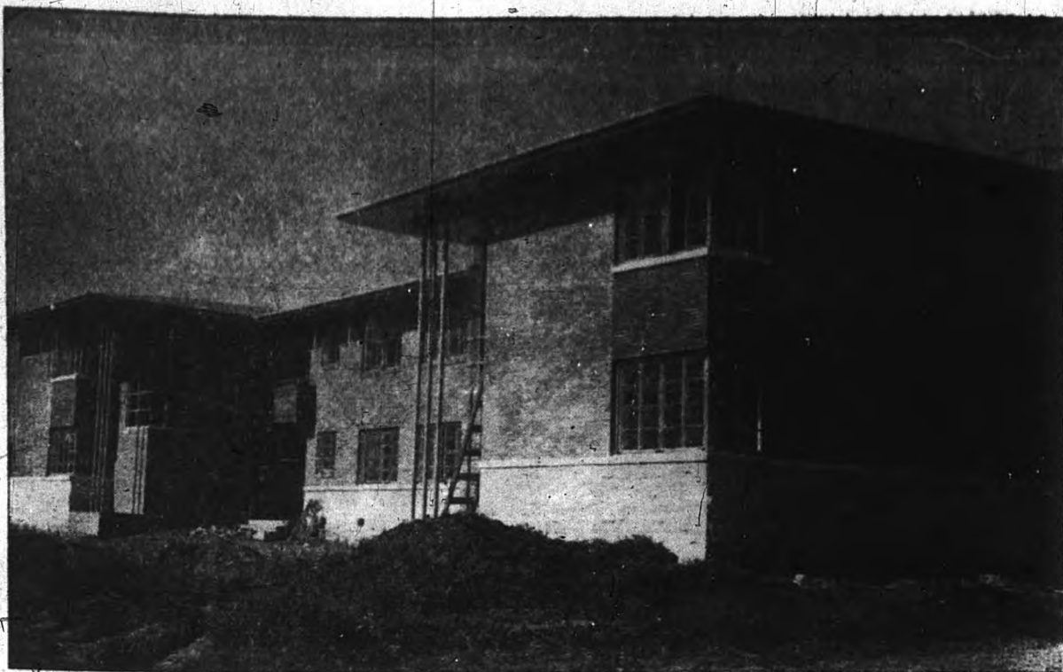
Here is a corner view of the new Hillcrest Apartments, located on South College Road, which are opening this week. The picture was taken before landscaping was begun. A great deal of the construction work was done by local firms.
