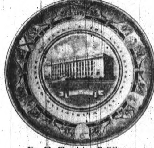
No. 12. Chemistry Building Erected 1933
