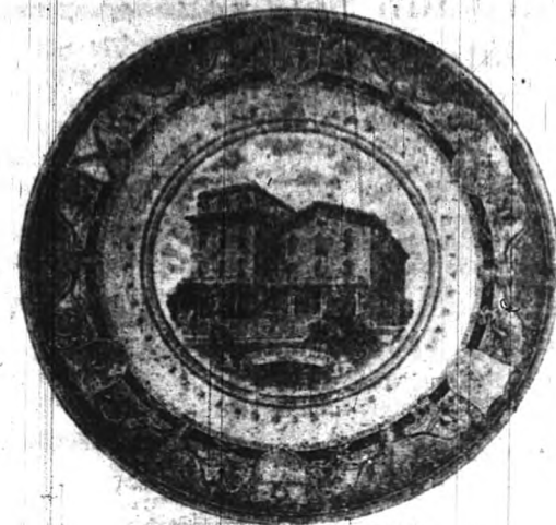
No. 1. Gathright Hall Erected 1876
