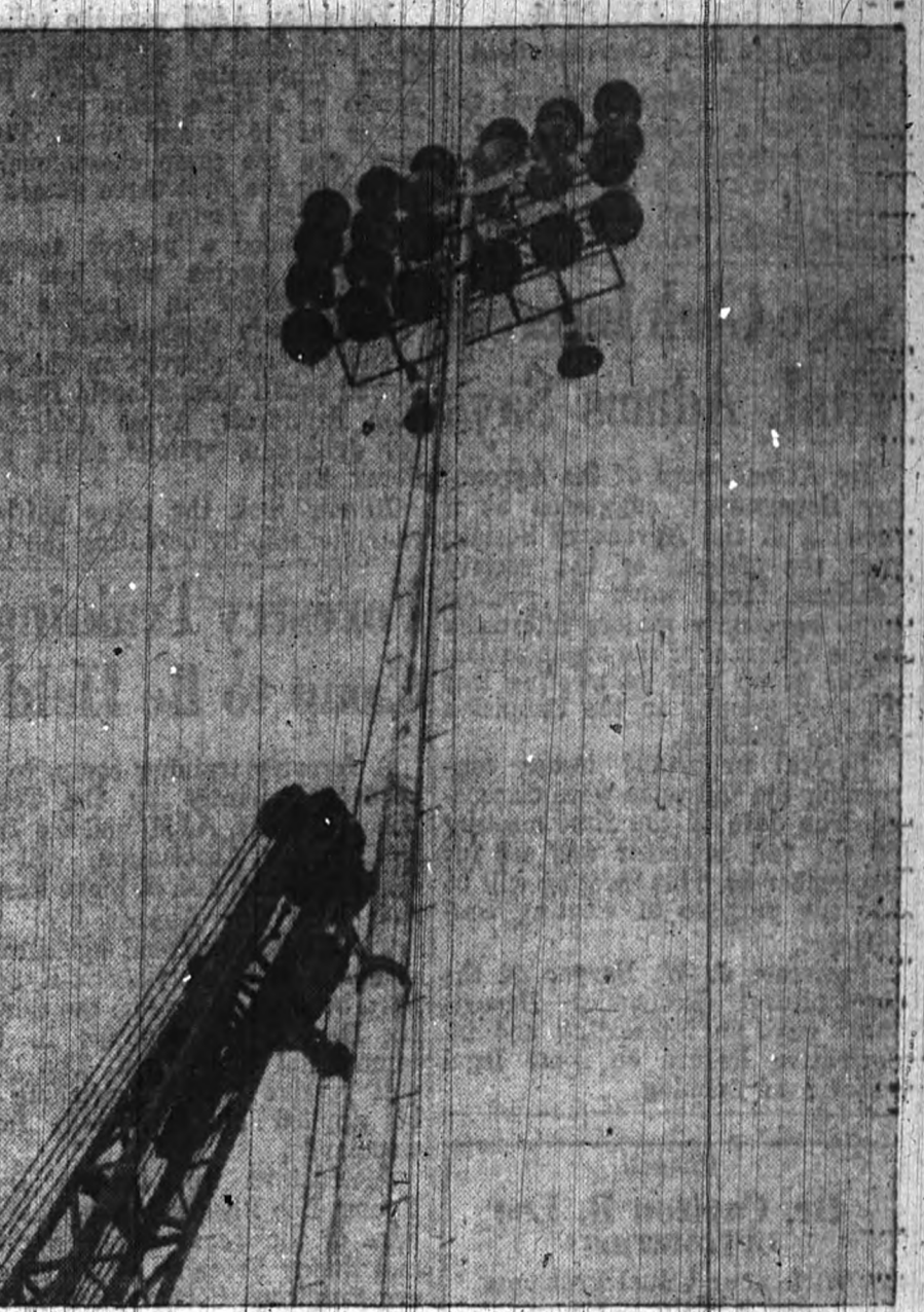
The Battalion photographer caught these workmen last week just as they were loosening the chain which was used to hoist the last steel post into place for the Kyle Field lighting system. The second workman can be seen behind the crane boom. The Farnsworth and Chambers Construction Co., which erected the poles, used a crane with a 75 foot boom for the job.
