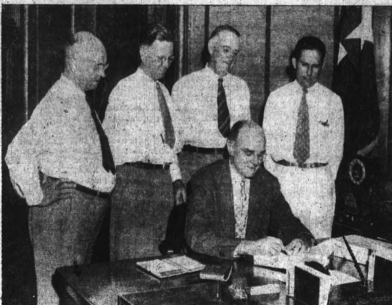
CHANCELLOR GIBB GILCHRIST signs the contract for the McKee Company to begin construction on the Memorial Student Center. Onlookers from left to right are T. R. SPENCE, E. E. McQUILLEN, C. W. ADAMS, and DICK HERVEY.
