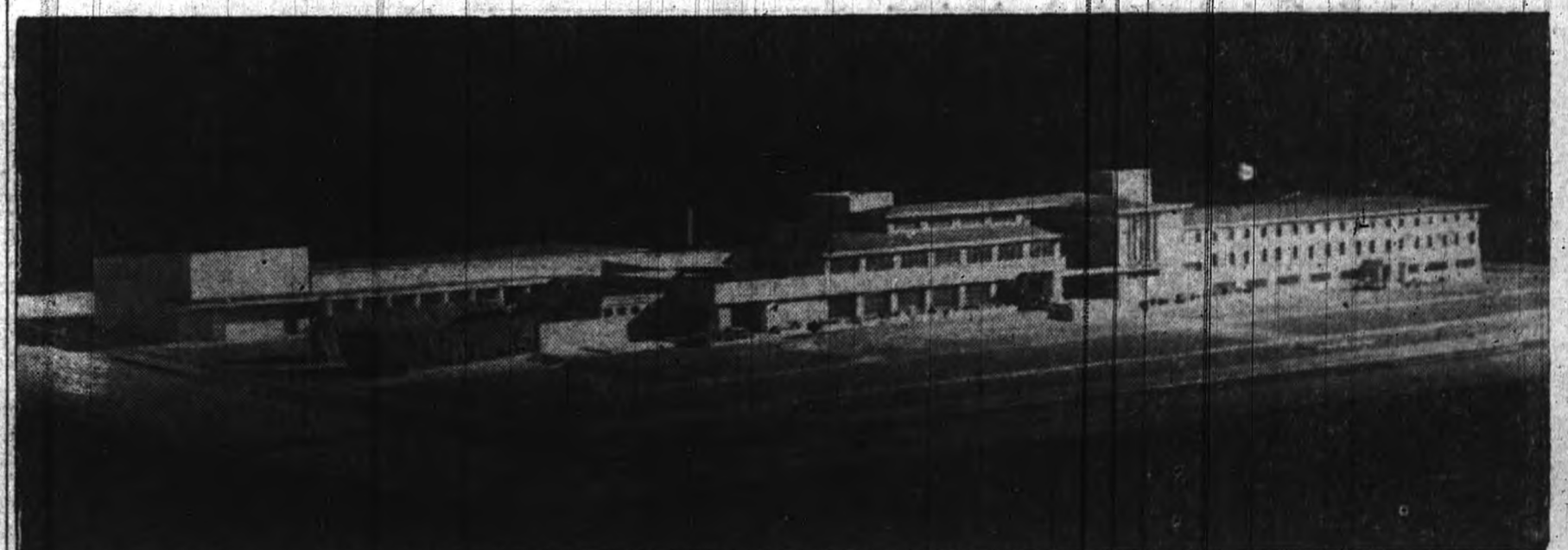
STUDENT MEMORIAL CENTER MODEL. The three units for which bids have been submitted will make up the heart of the Center. UNIT 1 will contain four food services, dining room, coffee shop, fountain, barber shop, gift shop, post office, dancing terrace, dark room, workshop, and main desk for the hotel. UNIT 2 will include 64 hotel rooms, four large rooms, long distance telephone center, browsing room, trophy case, Student Senate Chamber, and offices. UNIT 3 will be made up of eight bowling alleys and 12 billiard tables.
