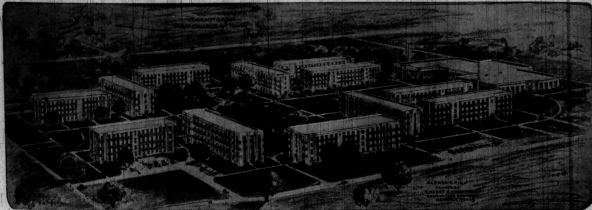
Shown above is the new housing unit for A. & M., composed of 12 new dormitories and a new mess hall. Construction is scheduled to be completed in time for occupancy the first of next year.
