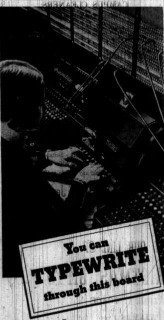
It looks like a telephone switchboard actually it's a Teletypewriter exchange switchboard. Through such boards-located in 160 cities and townsalready more than 11,000 subscribers to Teletypewriter service are being inter-connected.
