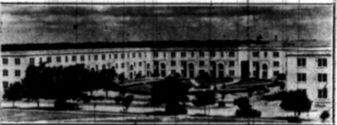
Law and Puryear Halls, erected in 1928. These two dormitories face each other on an open court. They contain 168 rooms each and are equipped with the most modern in heating and ventilating systems. These buildings are built on the ramp system and have separate shower and toilet facilities for each four rooms.
