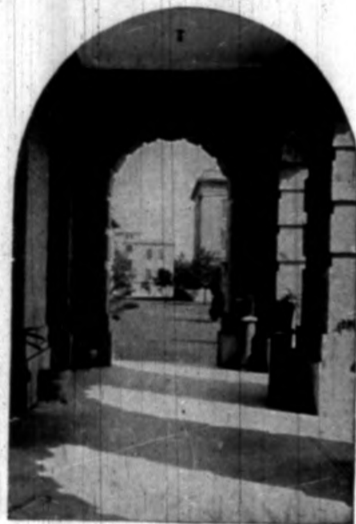
LOOKING SOUTH FROM EN- TRANCE OF ACADEMIC BUILDING
