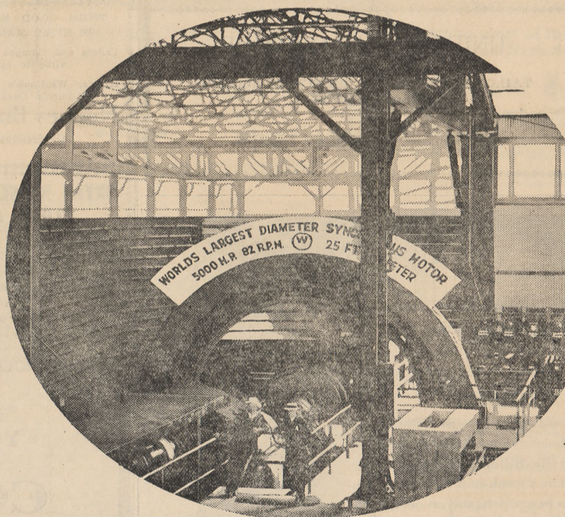
This 5,000 h. p. motor in the Columbia Steel Company's plant, with its frame of arc-welded steel, is physically the largest synchronous motor ever built.
