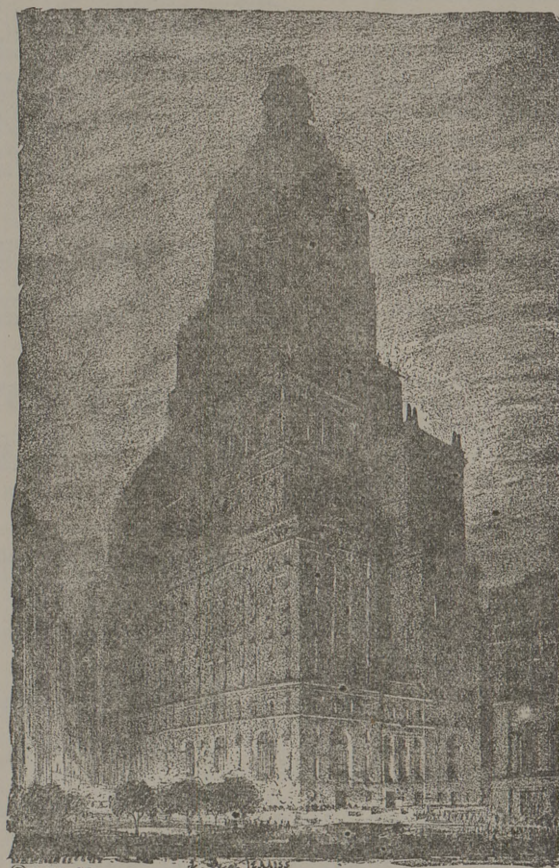
The Complete Project for the Standard Oil Building New York City CARRÉRE and HASTINGS Architects
