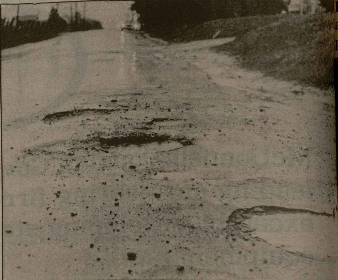
These chuck holes at Holleman and Welsh streets are just a few in College Station that are badly in need of repair. Federal government funds will repair streets in low income areas of College Station. Battalion photo by Kayce Giam
