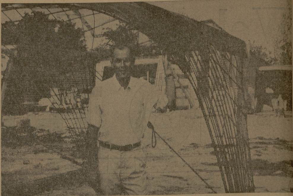
Examining steel reinforcing rods are arched to the desired shape with the use of steel cables in the second stage of construction of his new process.
