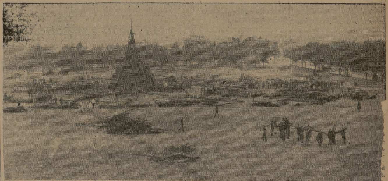
Hundreds of students gather on the Main drill field Sunday afternoon to take part in building the biggest bonfire in A&M's history. Already 10 feet taller than last year's bonfire, the center pole measures 65 feet. Scattered around the base are logs, which were hauled in from the cutting areas Sunday. When this picture was taken late Sunday afternoon, the biggest portion of the days
